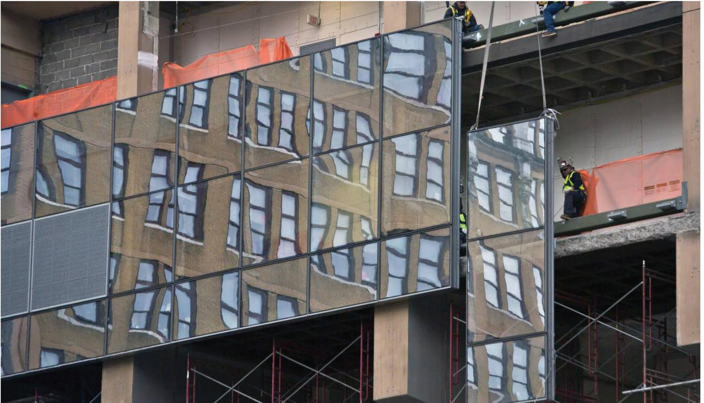
A typical high-rise office tower can need hundreds of thousands of square feet of metal-framed glass panels. A Brookfield Property under construction in New York
