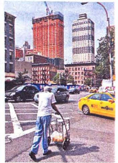
Construction on 42nd St. towers over the highly trafficked area
